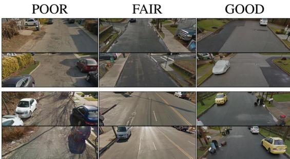
Figure 3: **Examples of pavement images.** For each condition, two street segments are shown, each with two images. Images were cropped from the original  $640 \times 640$  images.
