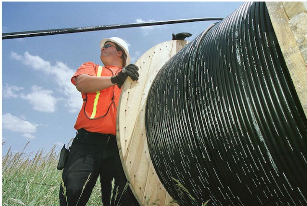
Damage to Spectrum's fiberoptic cables led to widespread internet loss throughout Queens and Brooklyn this morning. (Getty Images)
