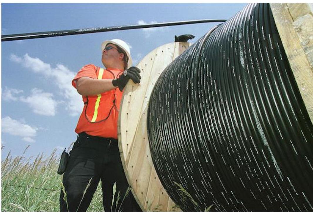
Damage to Spectrum's fiberoptic cables led to widespread internet loss throughout Queens and Brooklyn this morning. (Getty Images)
